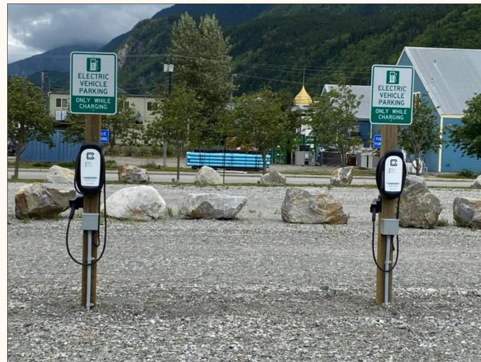
Level 2 EV chargers near the public works building in Skagway, Alaska.
